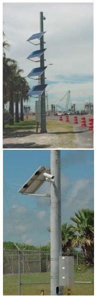
12VDC.) The pan-tilt-zoom cameras all have heaters to prevent condensation with cool weather as well as maintain a minimum temperature when it becomes cold.
